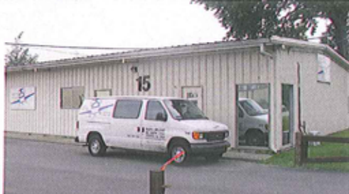
Stationed directly on the field at HPN, Rudy's White Plains facility services airport locations such as FRG, HPN, ISP, JFK, LGA and SWF for around-the-clock service.
